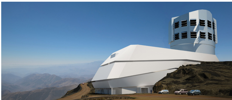
Current LSST summit facility design concept is shaped by wind and topography
